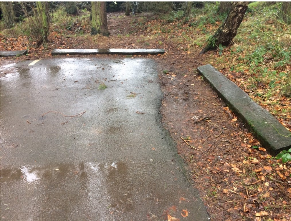
Figure 2 Damaged edging replacements and full bay lining required
