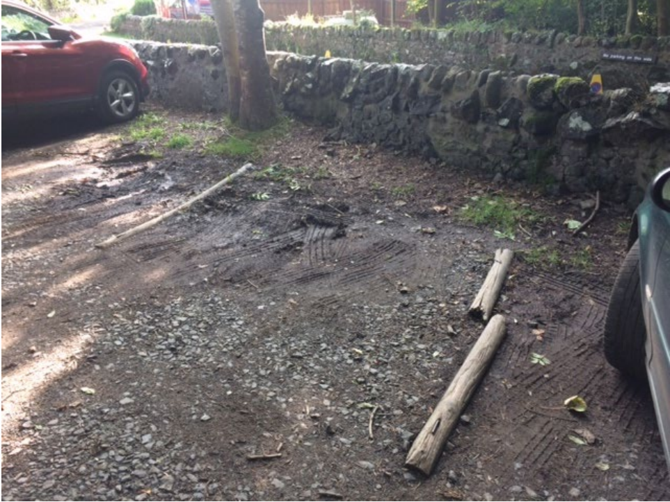
Figure 3-4 damaged space markers and insufficient tarring in car park
