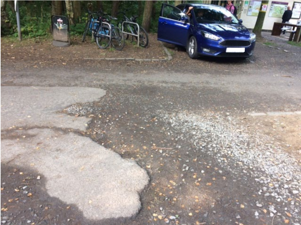
Figure 3-4 damaged space markers and insufficient tarring in car park
