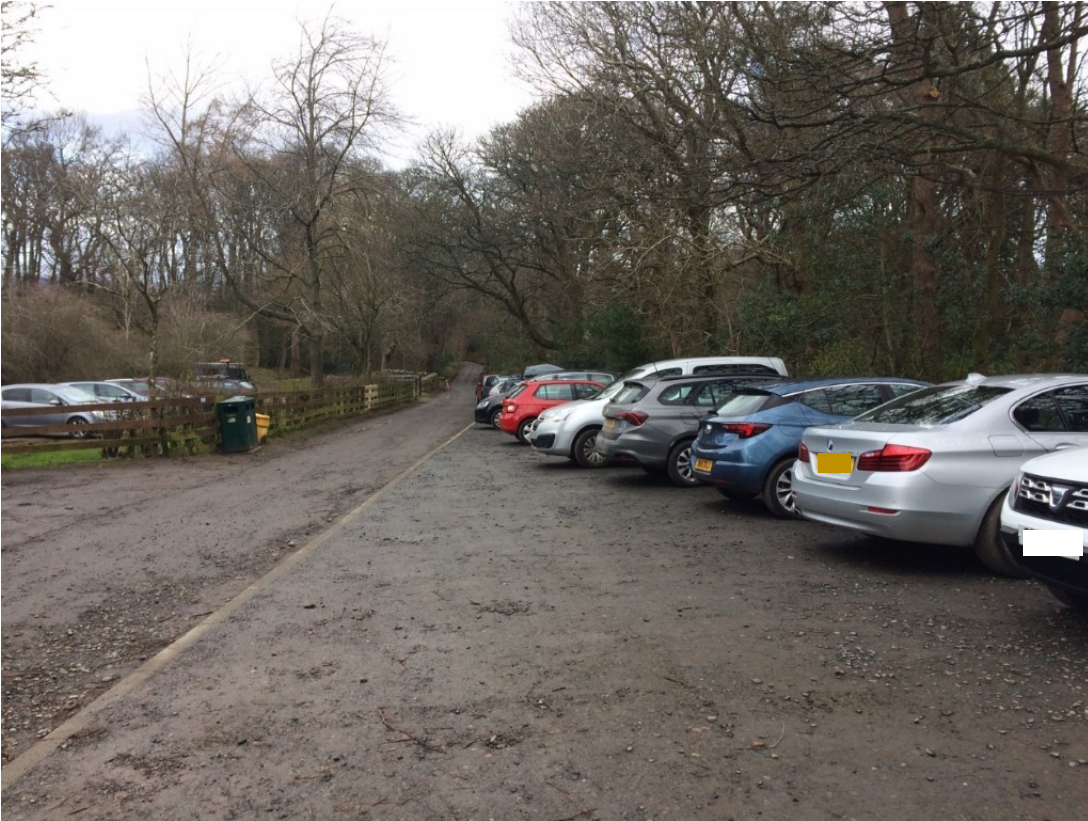
Figure 5 No parking bay delineation or appropriate turning area
